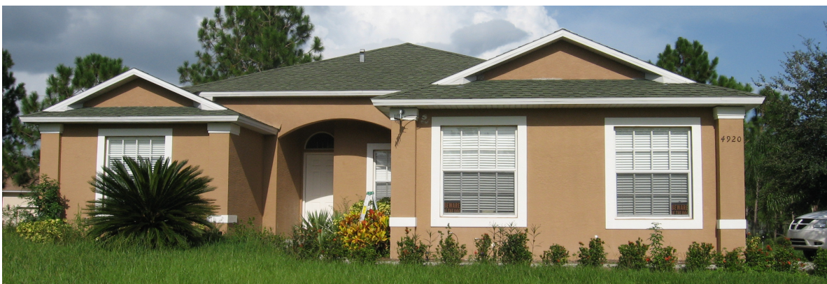
Figure 1-1 - Photograph of west face of house in Naples, FL
